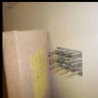
Glue or screw impaling clip to the wall and allow to dry completely.
