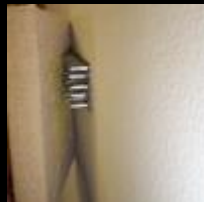
Align panel and impaling clips so that impaling clip touches the fiberglass rather than the fabric wrapped around the back of the panel.
