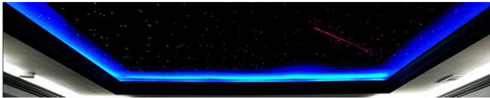
Accent lighting installed on your own molding under the star panel area perimeter
